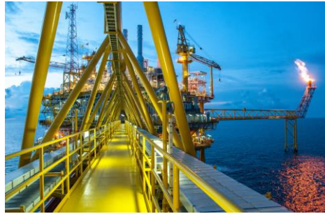
Protection of High-Risk Installations
