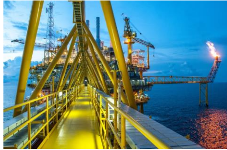
Protection of High-Risk Installations
